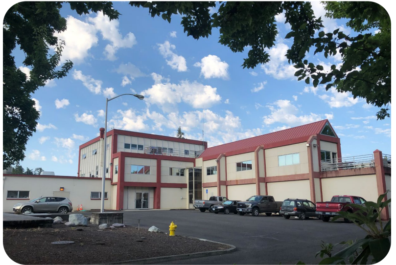
The CRW treatment plant has been in operation since 1964.
