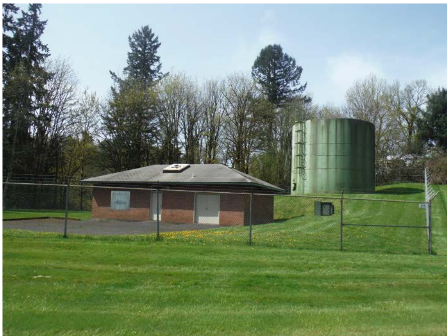
Photo 1: Well No. 1 Pump Station and Reservoir, looking north (April 9, 2018).
